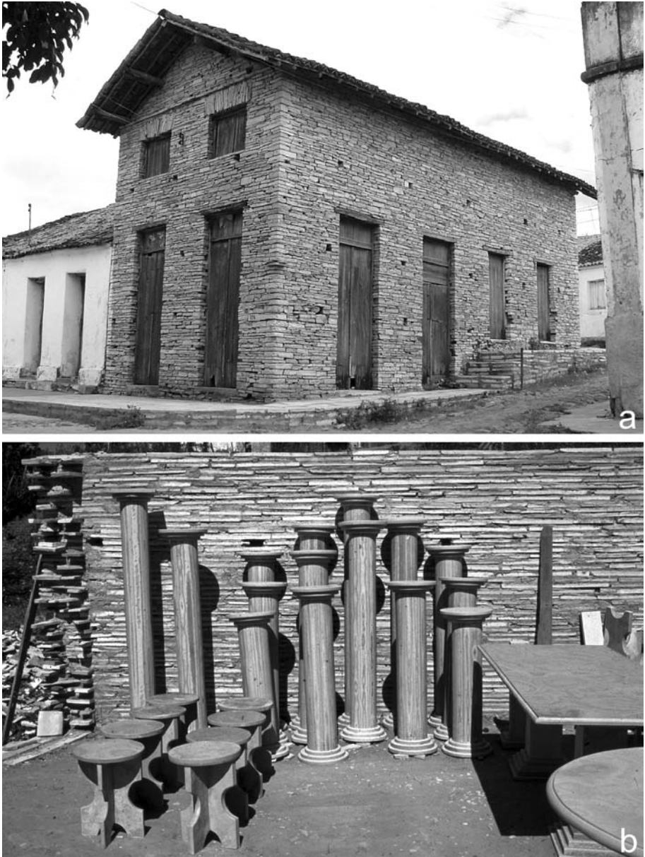
Fig. 5.3. Economic uses of the Nova Olinda Member limestone. (a) Historically used as building stone, Araraporanga, Ceará. (b) Ornamental use of unweathered stone for tables and 'neo-classical' columns, manufactured by Sr Anton Filipe, Nova Olinda.
