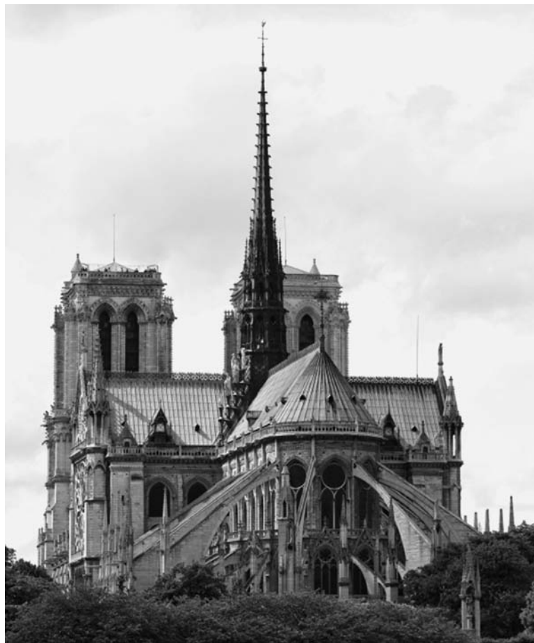
Figure 8.15 Flying buttresses. These struts help support the walls of large gothic cathedrals. Shown are examples from: (a) the Cathedral of Jerez de la Frontera in Andalusia, Spain © S. Morris; (b) the backside of Notre Dame Cathedral © J. L. Gutierrez. Both images from iStockPhoto.com.
