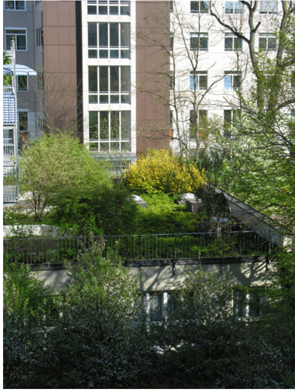
Fig. 6.1 In the absence of large urban green spaces constructed plant assemblages, such green roofs contribute to human well-being, as well as maintaining higher biodiversity. (Photo was taken in Munich, Germany by K Szlavecz)
