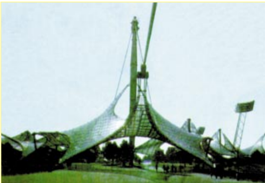
The roof of the Munich Olympic Stadium was inspired by spider webs. In this way the various tensions are evenly distributed over the roof.
