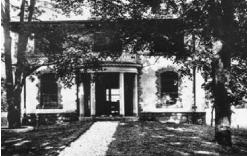
The building used for the Eugenics Record Office was located just north of the Cold Spring Harbor Laboratory. (Courtesy of CSHL Archives.)
