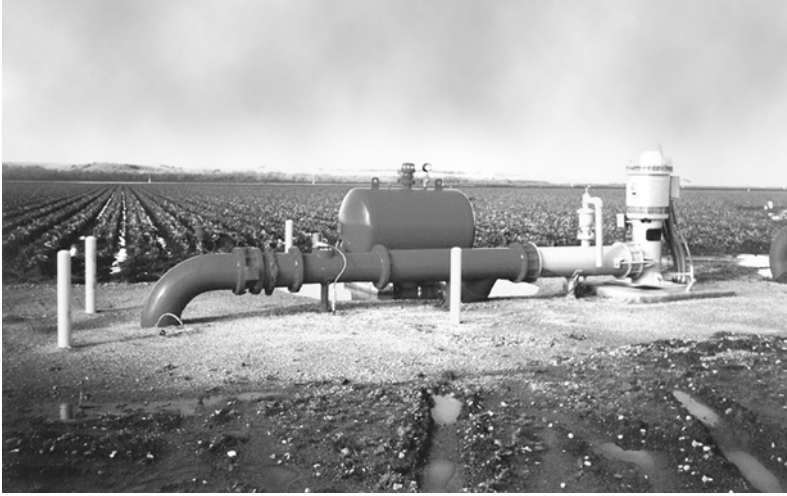
Figure 12.3.3 View of the irrigated area in Monterey County: recycled water is blended with well water to ensure adequate supply during peak summer months when demand cannot be met by recycled water supply alone.
