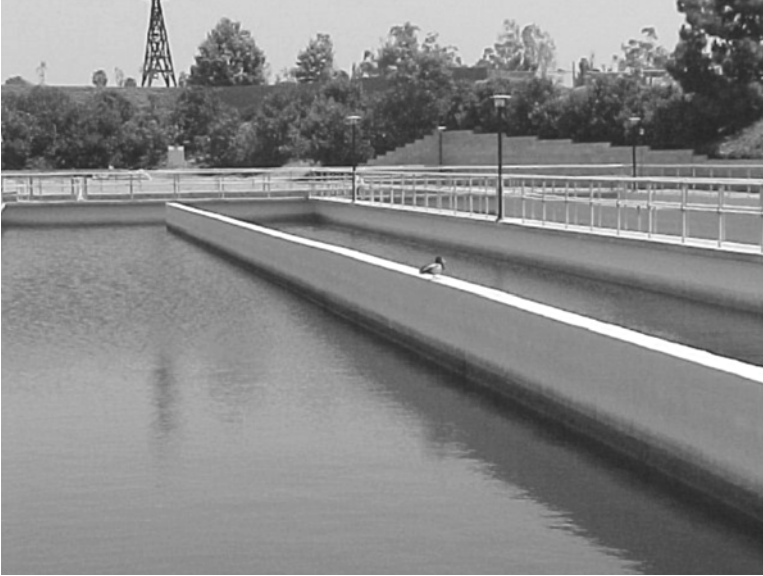
Figure 7.13 Plug-flow chlorine-contact basins in Irvine Ranch, California (agricultural and landscape irrigation).
