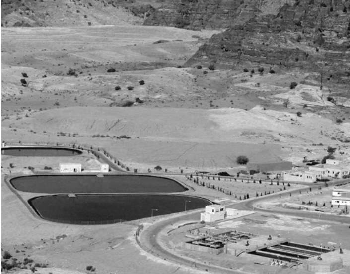
Figure 7.6 Maturation ponds at the treatment plant Wadi Mousa near Petra, Jordan (agricultural irrigation).
