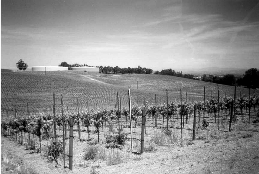
Figure 4.5 View of closed storage reservoirs in Santa Rosa, California, implemented for irrigation of vineyards.
