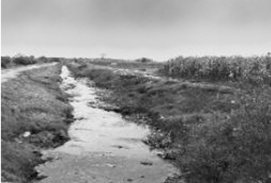
Figure 12.1.11 Unlined channel used to transport wastewater for irrigation in the Mezquital Valley.
