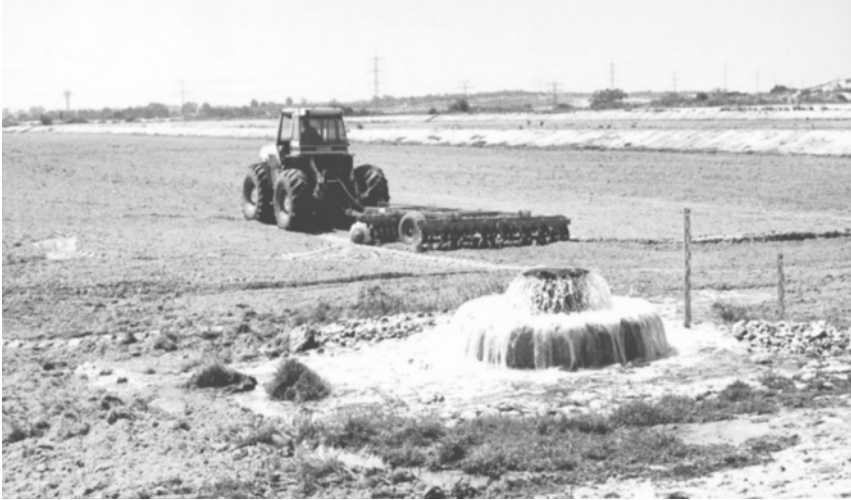
Figure 7.10 A recharge basin at the beginning of the filling cycle and a soil treatment machine: the Dan Region recycling plant, Israel (agricultural irrigation).
