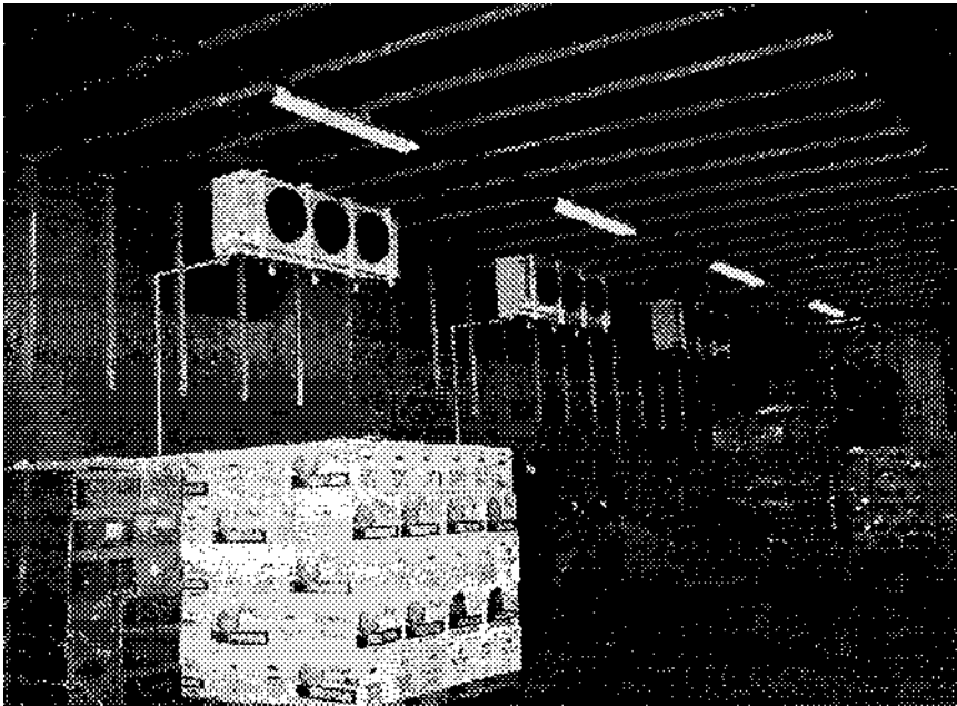
Fig. 6 Refrigerated storage room cooled by mechanical refrigeration.
