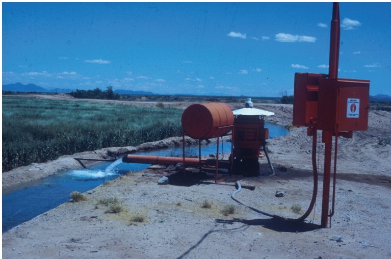
Fig. 5.6 Groundwater being pumped into a distribution canal
