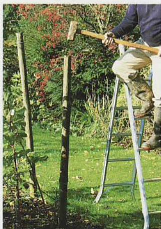
1 Using a large mallet, drive a strong wooden post into the ground at the end of a row of the fruit bushes to a depth of about 60cm (2ft).
