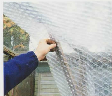
Above: Bubble-wrap plastic is an ideal material with which to insulate the greenhouse in the winter.
