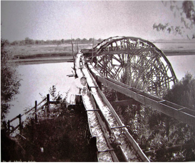
Fig. 4 Water Wheel lifting irrigation water at the river side in Adana (Ca. 1955)
