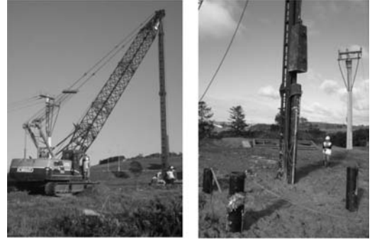
Figure 3. Pile driving at Albany, Auckland.
