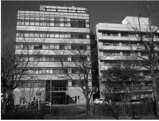
Figure 1. Front view of BRI annex building (left) and main building (right). These two buildings are connected by passage ways as seen in the picture.
