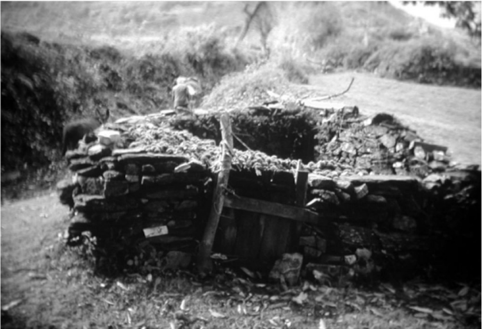
Figure 26. Small construction to store nuts into the burs in Galicia.
