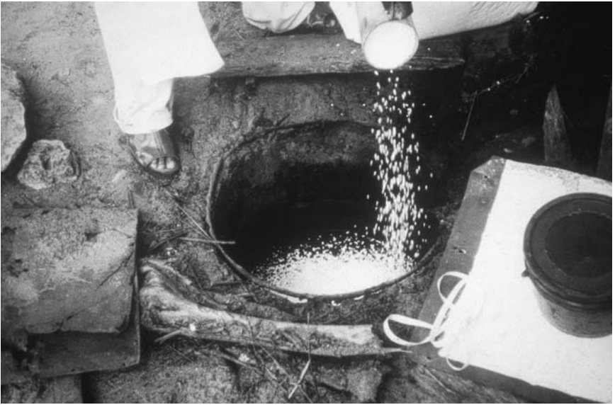
Fig. 12.2. Pouring expanded polystyrene beads down a soak-away pit to prevent colonisation by the mosquito, Culex quinquefasciatus (courtesy of C. F. Curtis).
