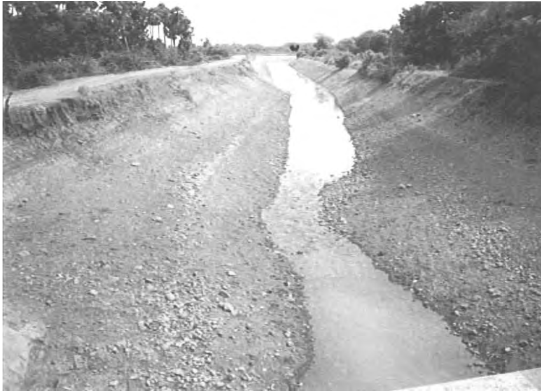
figure 6.2 Yeleru Left Bank Canal, a natural parabolic
