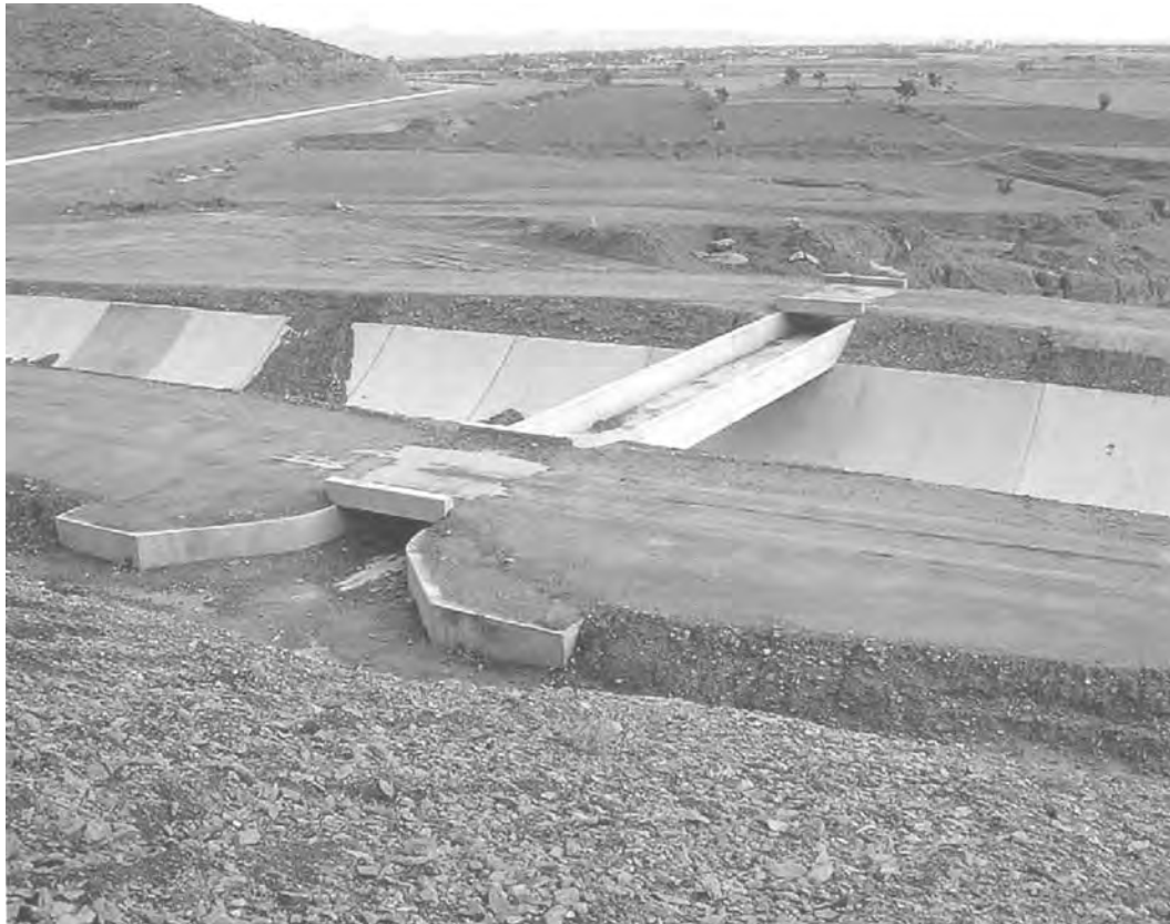
figure 7.19 Small superpassage on the Pehur High Level Canal, Pakistan
