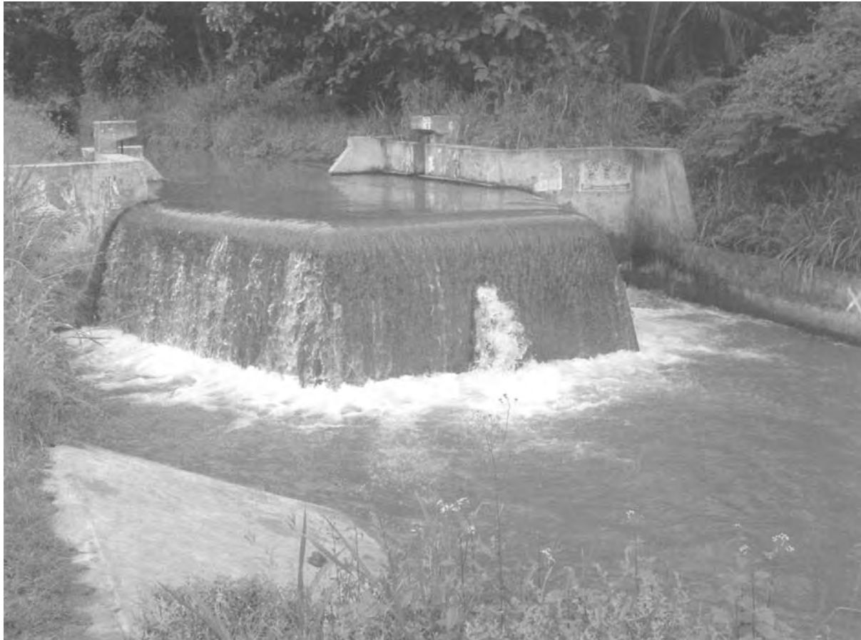
figure 7.10 A long-crested weir with convex duckbill configuration, Sri Lanka System H. The crest is round-nosed. This arrangement gives excellent energy dissipation. Note the drainage orifice in the centre
