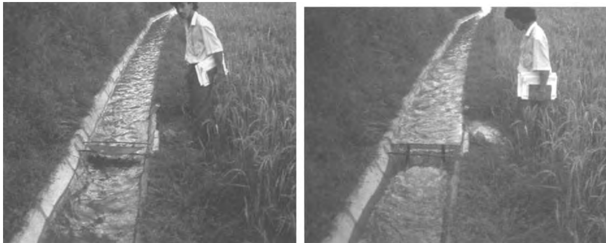
figure 7.11 Parabolic check plate, with field outlet closed at left, open at right
