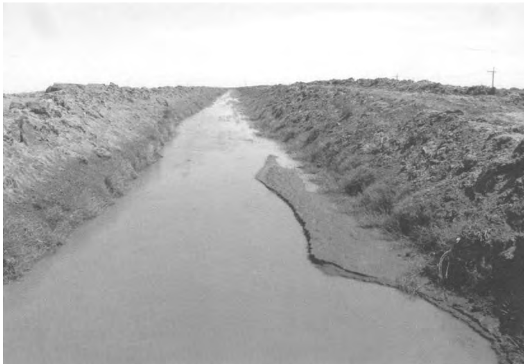
figure 4.6 Silt accumulating in a Gezira minor canal, Sudan. As the silt is dug out, the banks grow higher each year
