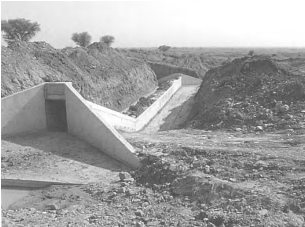
figure 7.18 Drop inlet culvert under construction
