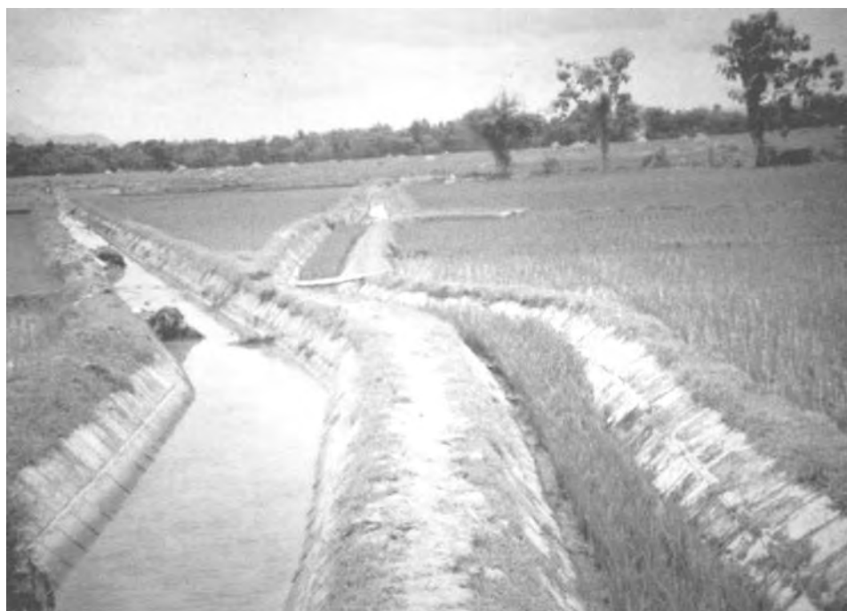
figure 11. 11 Redundant tertiary takes up useful land
