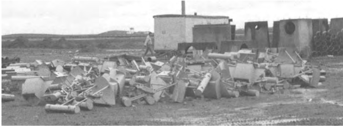
figure 4.11 Parabolic self-regulating upstream control gates awaiting installation, Maskane Project, Syria
