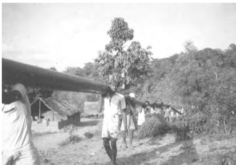
figure 8.7 Installing MDPE pipe, India
