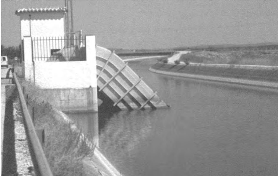
figure 7.22 A siphon side escape structure on the Genil-Cabra Canal, Spain
