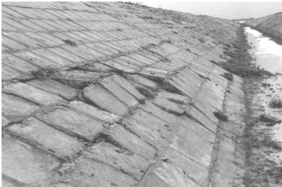
figure 9.5 Precast slabs sliding under their own weight, India.
