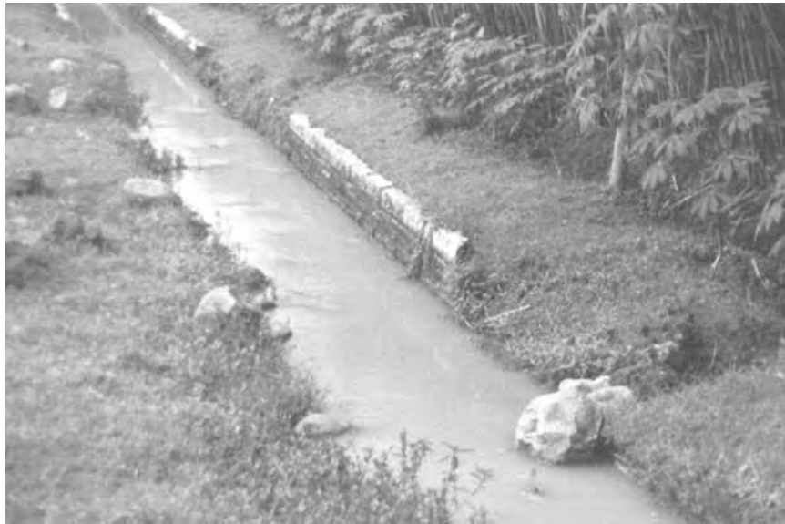
figure 6.8 In Eastern Java intensive land use means every available piece of soil is utilised. But cassava grown on canal banks soon destroys the lining
