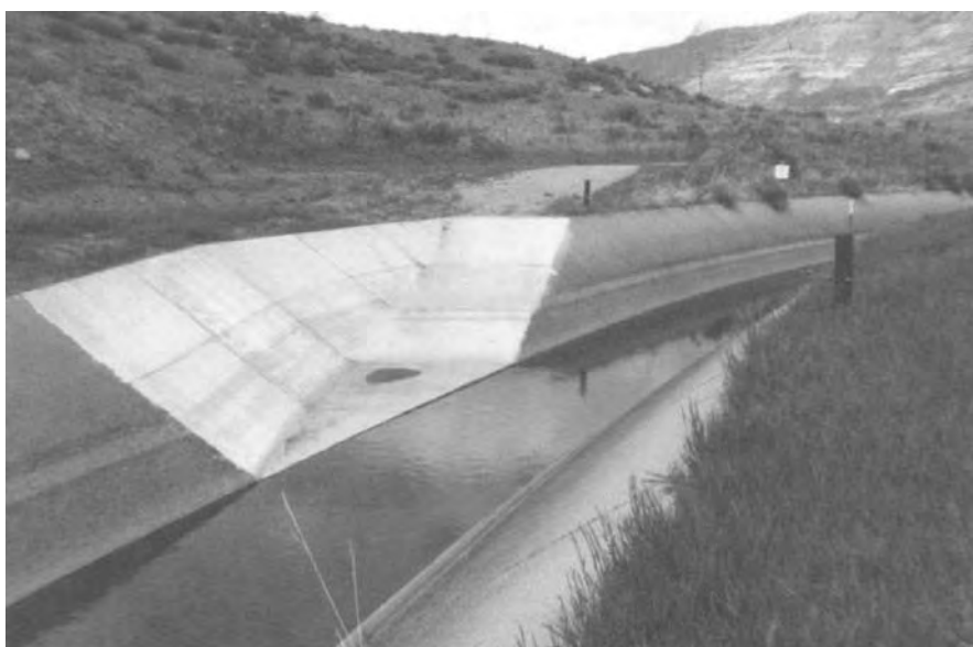
figure 7.1 An access ramp for canal maintenance, Colorado
