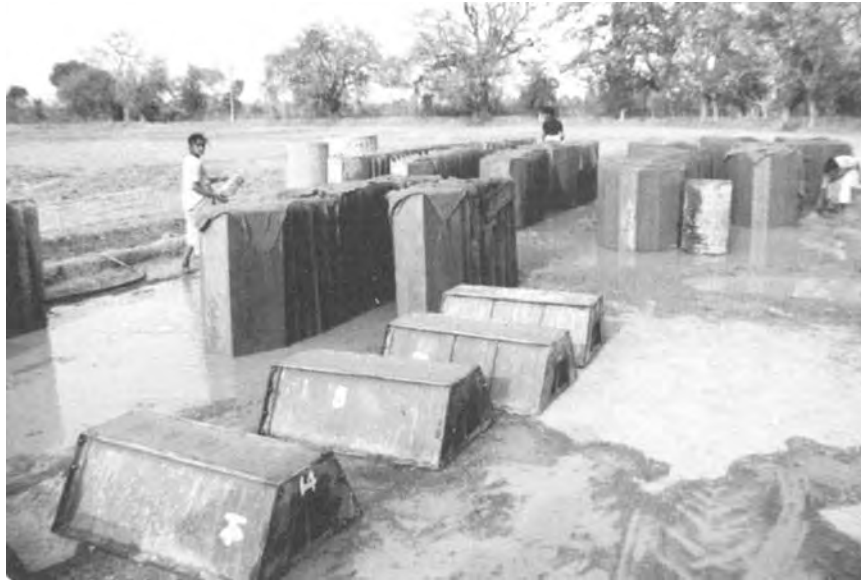
figure 9.12 A field casting yard for parabolics, India
