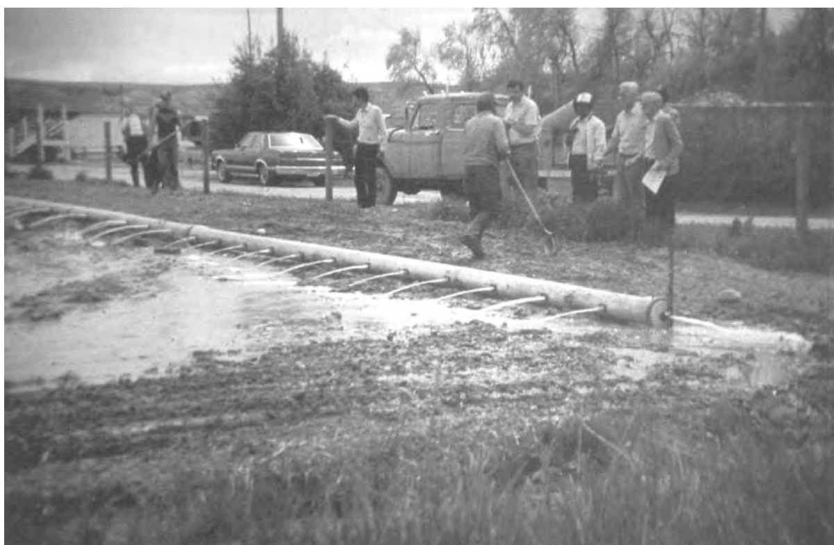
figure 8.6 Gated pipe system, USA
