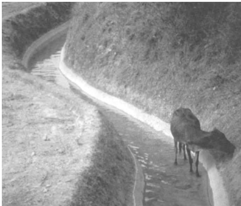
figure 6.9 Cattle can wreck small canals, especially in India where cows are sacred, and canals are not
