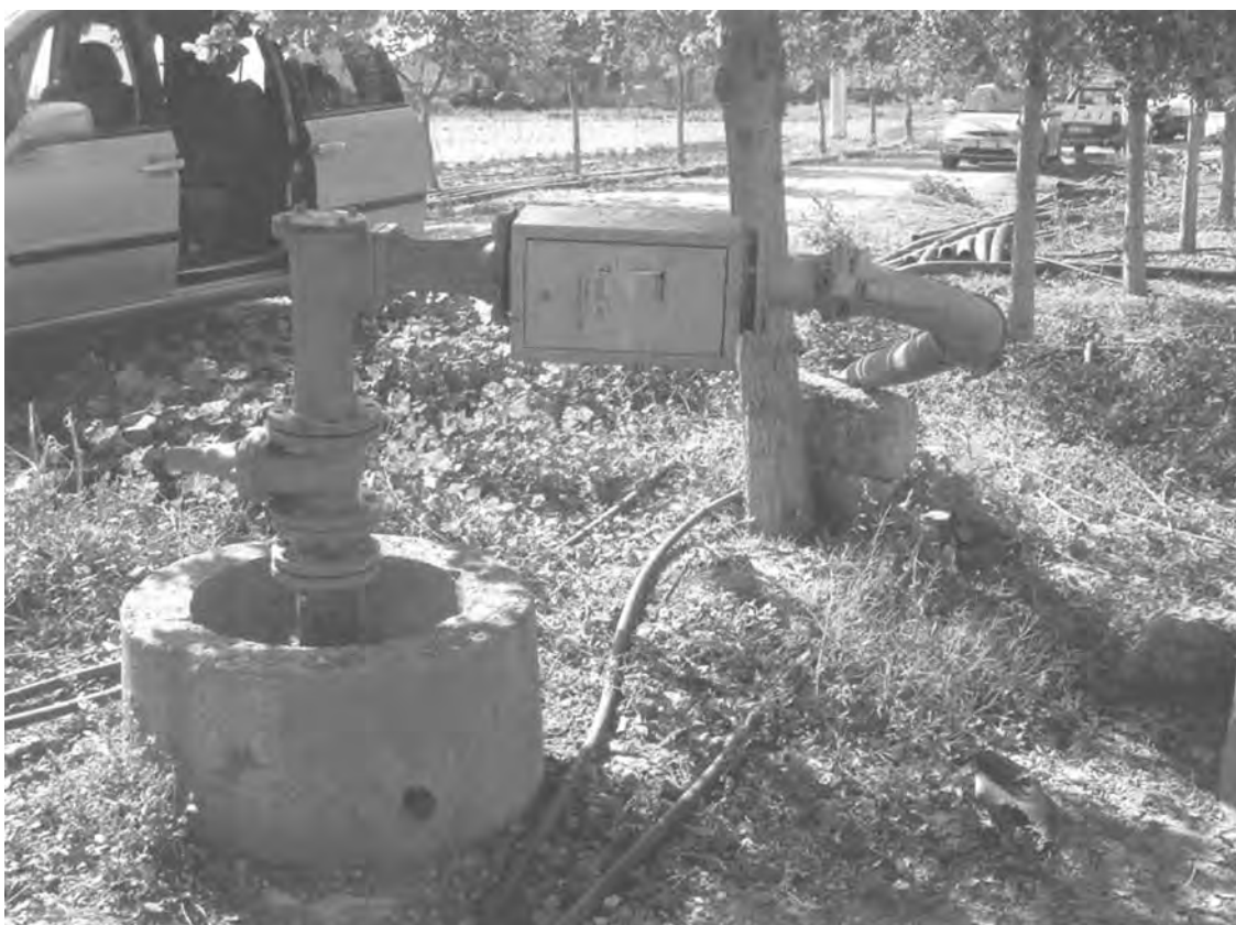
figure 3.11 an 'Acquacard' unit controlling water to a hectare of artichokes, Foggia, Italy
