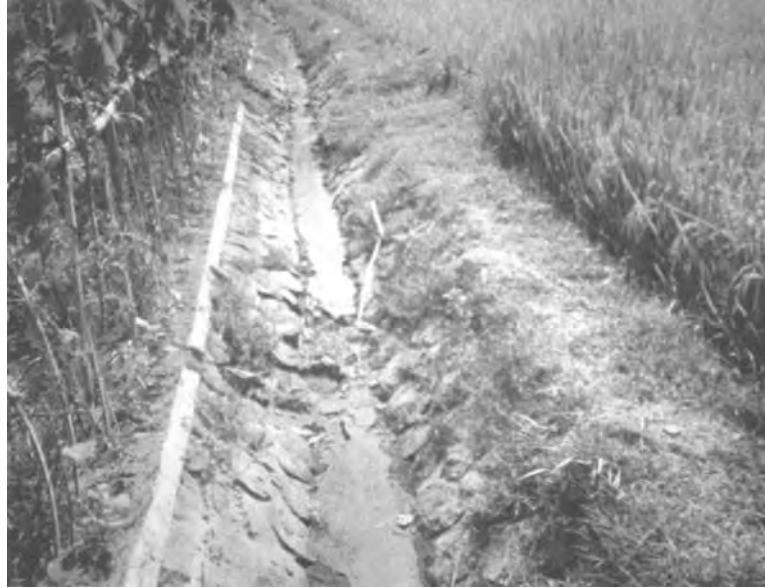
figure 11. 9 Crops on canal banks damage lining. Cassava, Java
