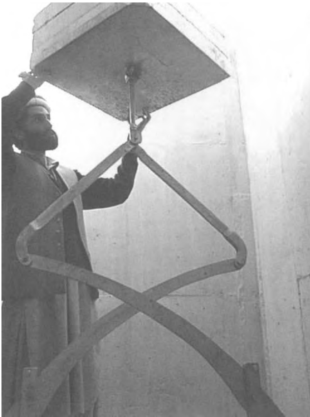
figure 8.10 Installing a Harris valve float
