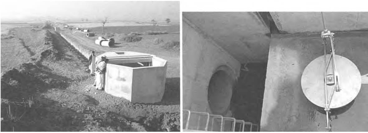
figure 8.9 Harris valve stands in Topi, Pakistan. These are very substantial structures, built to deter vandalism. These 24 inch diameter Harris valves are here arranged in pairs to handle the discharge of 1200 l/s
