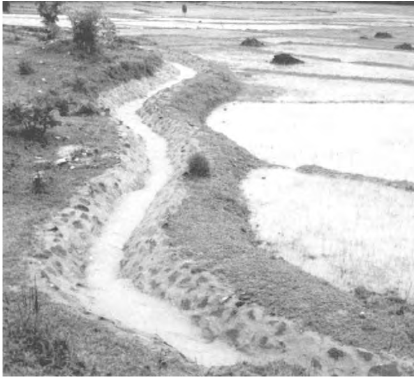
figure 9.3 Stone masonry, India
