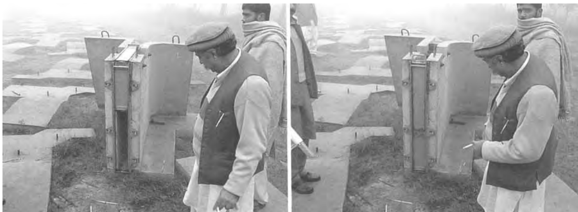
figure 4.8 Refusal gates installed on a precast outlet, Pakistan. (left – open, right – closed)
