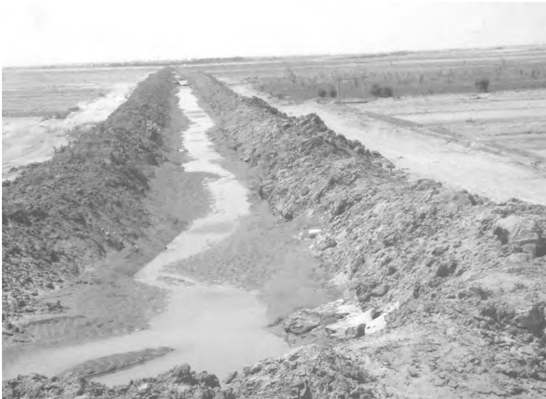
figure 5.6 Conditions leading to heavy water use. A hot, arid climate, persistent winds, sandy soils, poorly constructed canals and an inappropriate method of field irrigation. The Multaga project in Sudan
