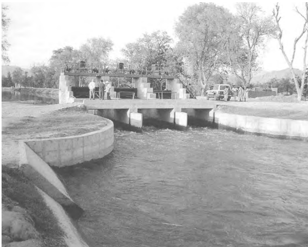
figure 3.6 Cross regulator on Machai Branch
