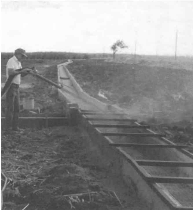
figure 9.10 Shotcreting a small canal, Swaziland (courtesy Chris Cronin)
