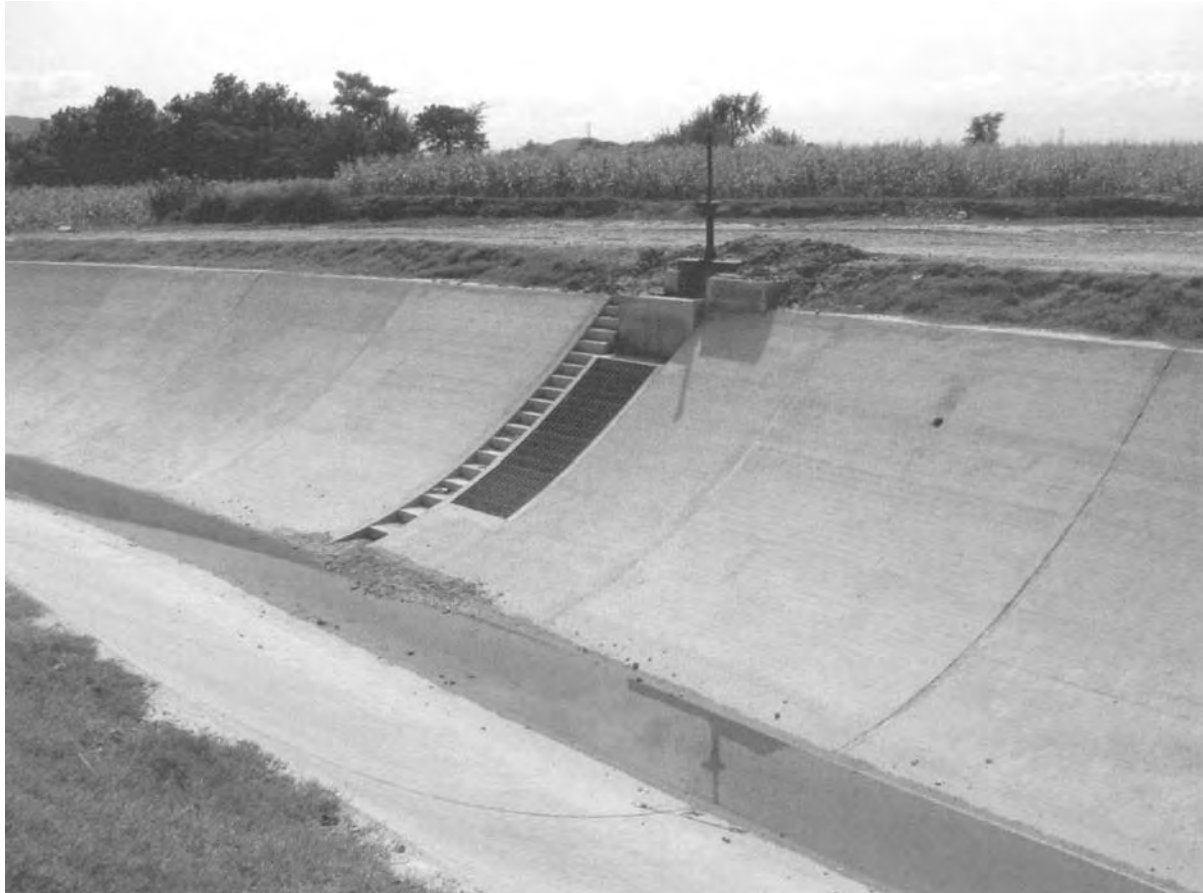
figure 8.14 Pipe intake from a level-top canal
