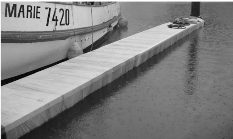
Fig. 14.4 A marina pontoon wrapped in geotextile fabric during efforts to control an infestation of the pest ascidian Didemnum vexillum in Tarakohe Harbour, New Zealand. Wrapping restricts water exchange to fouling communities growing on the pontoon, resulting in the development of anoxic conditions and eventual mortality. Photo: A. Coutts, Cawthron Institute.
