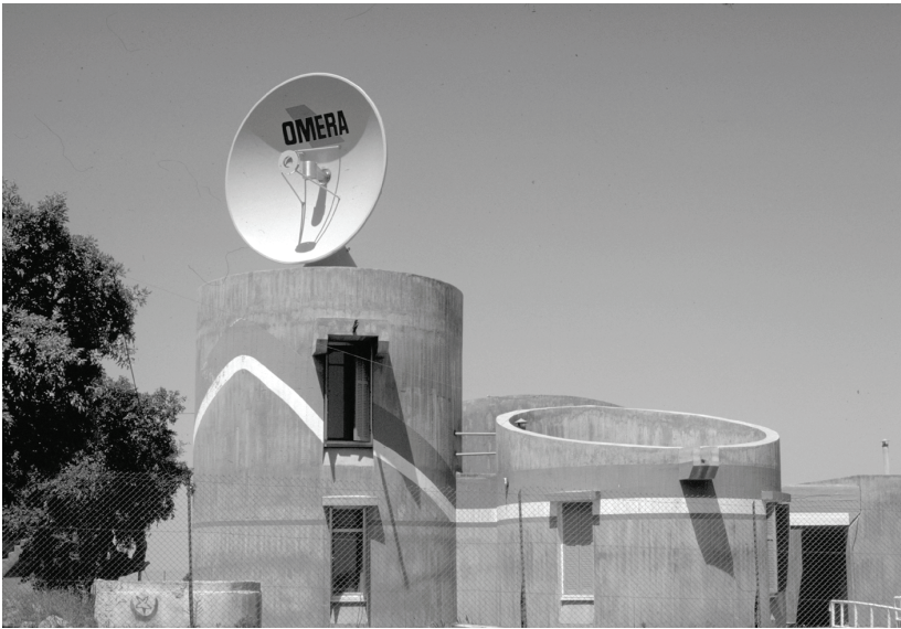
Fig. 8.5 : Meteorological radar (Tlemcen, Algeria).
