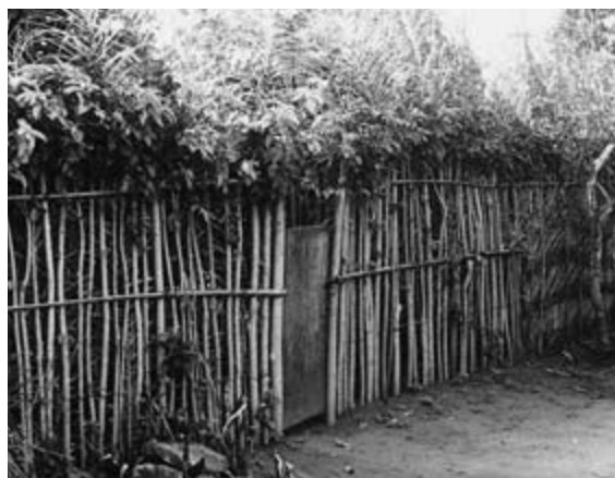
Figure 7.6 Yam barn in Nigeria showing the construction using live branches that produce leaves to provide a shaded humid environment.
