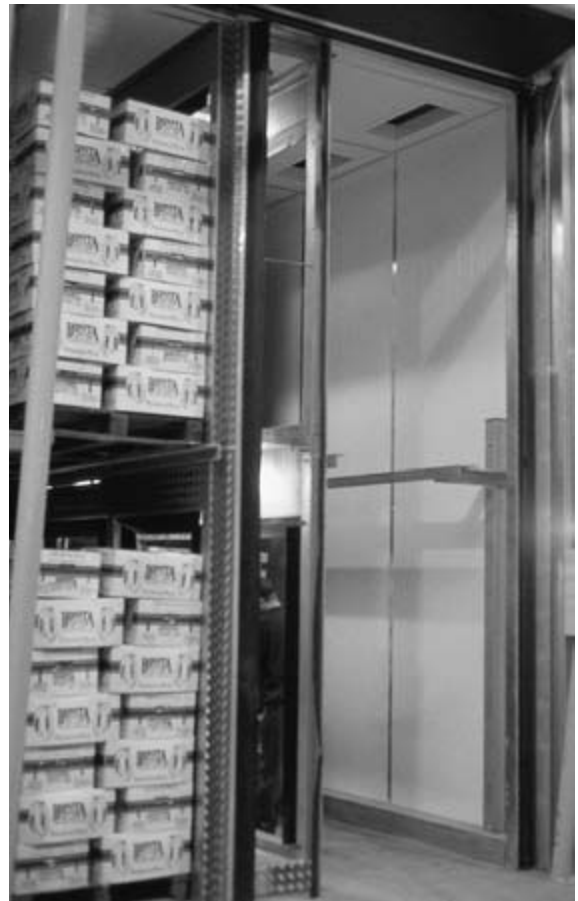
Figure 12.39 Pressure ripening room for bananas in Britain.
