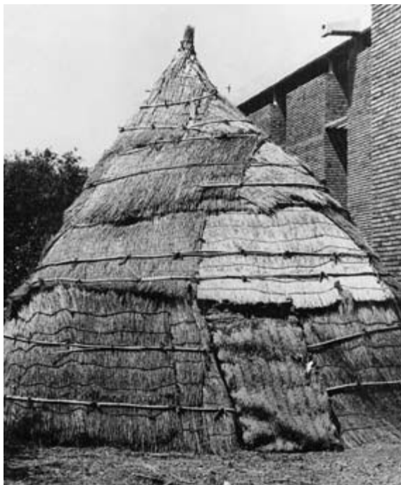
Figure 7.9 A traditional palm leaf store, called a rakuba, being used for onions in the Sudan. Source: Professor Sulafa Khalid Musa.
