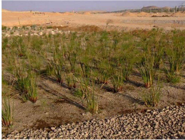
Figure 14.2: Wetlands constructed by the Neot Smadar Kibbutz, for ecologically friendly municipal and agricultural sewage treatment.
