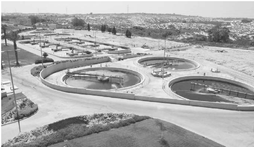
Figure 5.5: A view of the largest wastewater treatment plant in Israel.
