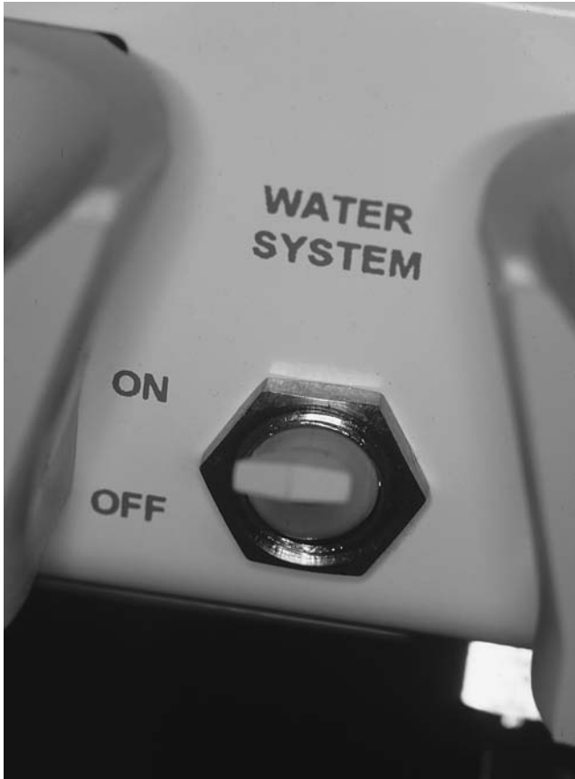
FIGURE 1.6. Most dental delivery systems have water on-off switches (iM3 pictured).
