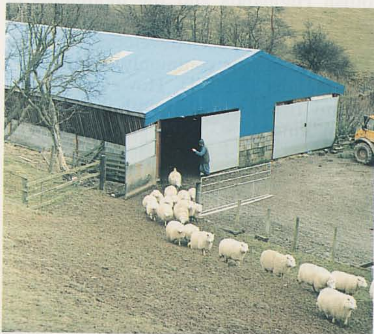
Fig. 7.2 Sheep shed typical of many erected on hill farms in the past 15 years.
