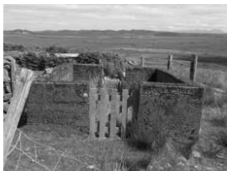
Fig. 7.28 Historic dippers such as this were often built close to watercourses, to facilitate filling. The dippers can no longer be used due to the high risk of groundwater contamination.
