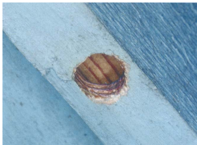
FIGURE 19.22 Circular entrance to nest of carpenter bee, Xylocopa virginica (Anthophoridae), in cedar wood of house eave. (Photo by G. R. Mullen.)
