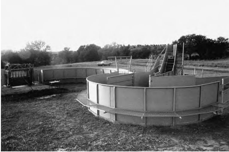
Fig. 7.5. The round crowd pen should have a completely solid fence and catwalk as shown. Some people prefer to remove the catwalk on the single-file race and work the animal's flight zone on the ground. In these systems, the fence on the outer radius of the single-file race is completely solid and the fence on the inner radius is solid only on the bottom half.
