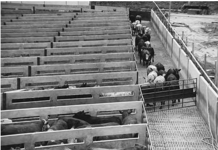
Fig. 20.3. Long, narrow pens on a 60° angle.
