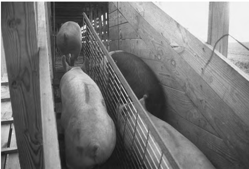
Fig. 14.3. A 'see-through' partition promotes following in this loading ramp. The outer fences are solid.
