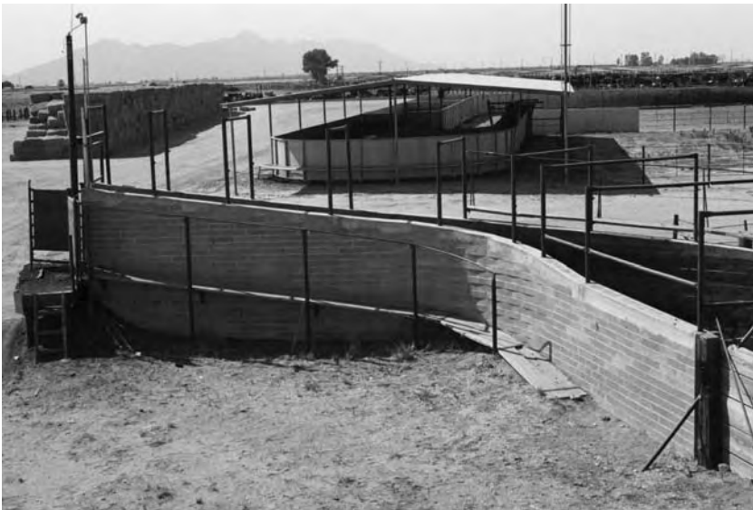
Fig. 1.1. Well-designed truck-loading ramp that could easily be constructed in a developing country by local people using readily available materials.
