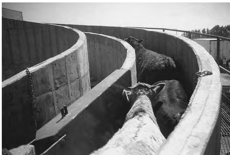
Fig. 20.5. Curved cattle race with solid sides at a slaughter plant; this design improves cattle movement.
