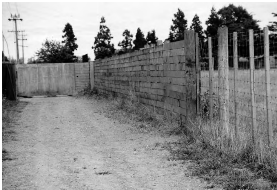
Fig. 17.1. Laneway fencing on approach to yards.
