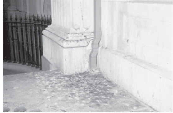
Figure 2.3 Bird droppings present dangers to humans, including slipping accidents and spread of pathogenic organisms.
