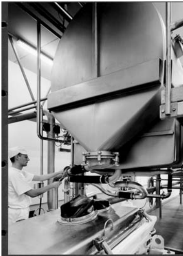
Fig. 3.21 Preparing the Vibro-Fluidizer ® for cleaning-in-place (CIP) by placing a funnel which returns the cleaning liquid to the CIP station. Data by permission of A.J. Partridge (personal communication) and GEA Process Engineering (Niro A/S), Gladsaxevej 305, Soeborg, Denmark.
