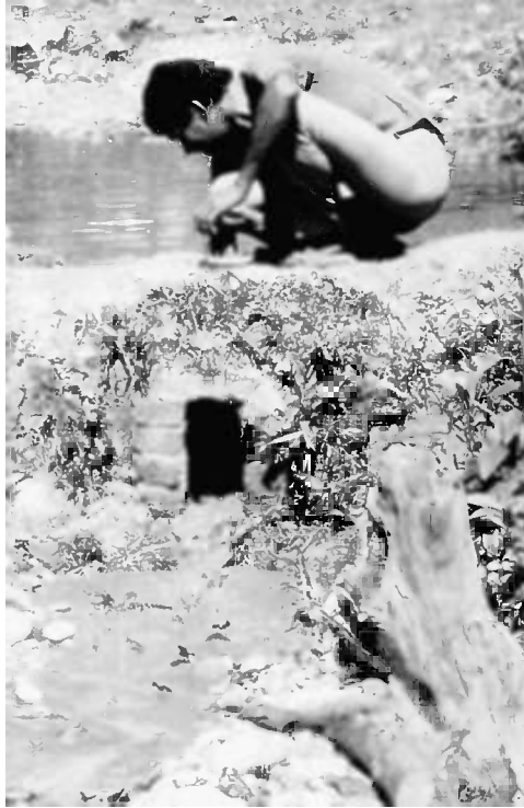
Fig. 3.11. A locally constructed dam for the control of Anopheles fluviatilis in Nepal. Every 3 days, the bung is removed and the head of water rushing down the stream is sufficient to dislodge developing mosquitoes.
