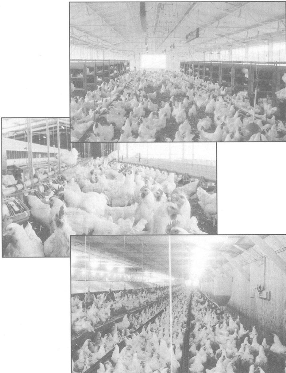
Fig. 8.9 Interior design for (Top) open-sided curtain (Middle) tunnel ventilated and (Bottom) fully controlled environment breeder houses. (Campi, Mexico; Fleming chicks, Ontario)
