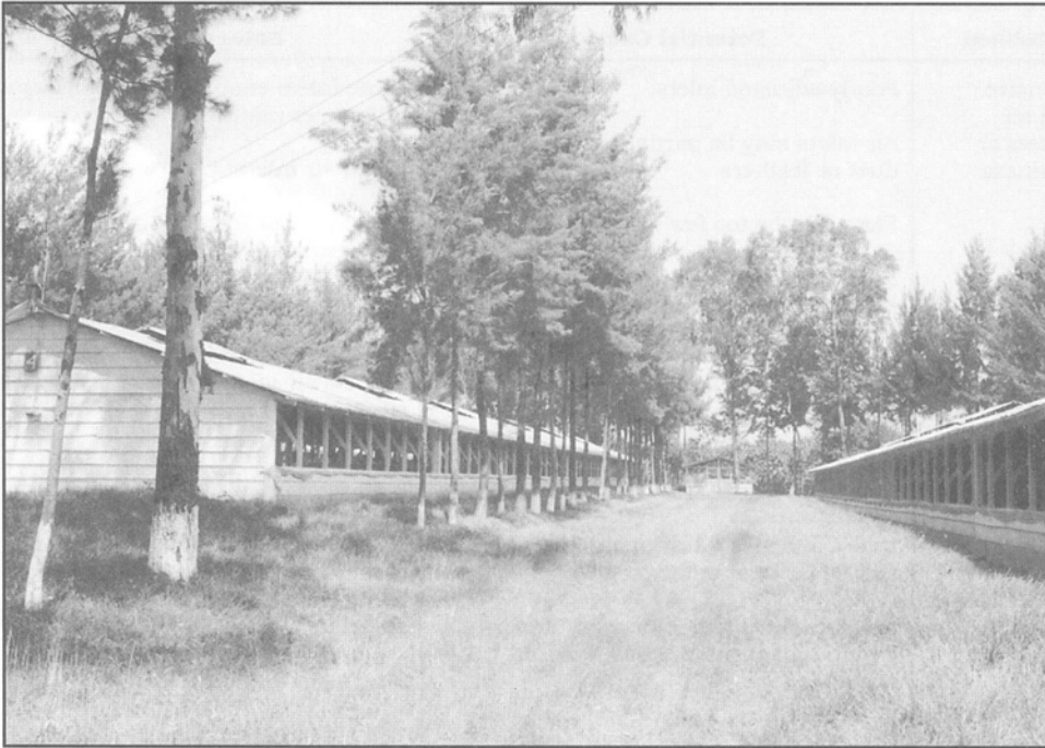
Fig 6.5 Shading from trees, with minimal disturbance to air flow (Avicola Villalobos, Guatemala)
