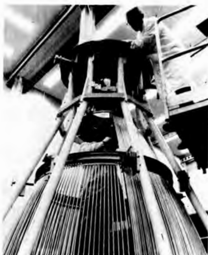
The J-2 liquid-hydrogen-fueled engine: statistics are presented at top left; at top right, the J-2's injector; above, left, a schematic of the J-2 engine systems; above, Rocketdyne workmen in a "clean room" in the Canoga Park plant are stacking the coolant tubes that will form the wall of a J-2 engine thrust chamber; at left, final assembly of J-2 engines at Canoga Park—J-2s for both the Saturn IB and the Saturn V; below, left, engineers study a J-2 engine that has simulated frigid space conditions; below, right, a cluster of five J-2 engines are readied for firing at Santa Susanna.
