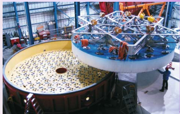
■ Below: Moving the 8.4-m primary with the vacuum lifting fixture from its shipping container into its cell in the mountain high bay staging area. The bell jar for aluminizing the mirror is the darker red structure hanging vertically in the upper right.
