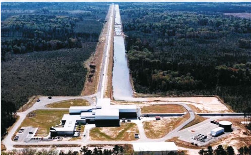
■ Left: The location of the two LIGO sites in the USA and aerial photographs of the LIGO installations in Hanford, WA ( middle ) and Livingston, LA ( bottom ).
