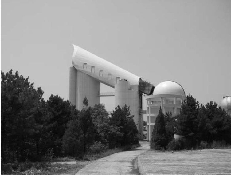
Fig. 11.2 The 4-m LAMOST Schmidt-type wide-field telescope. The primary mirror is housed in the dome to the right. The primary sends the light to a large stationary reflecting Schmidt corrector, which is located at the upper end of the inclined enclosure to the left. The focal plane (with a 5 degree field of view) is near the lower end of the inclined enclosure. (Photo Courtesy Norbert Christlieb)
