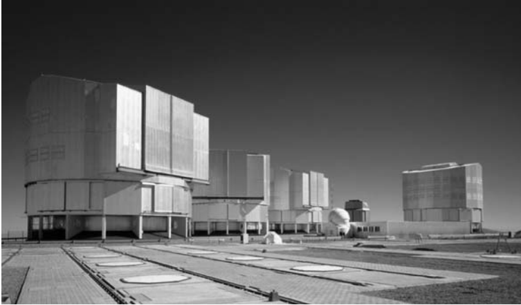
Fig. 4.5 The Very Large Telescope of the European Southern Observatory. The VLT consists of four large (8.2 m aperture) stationary telescopes and four smaller (1.8-m aperture) movable “auxiliary” telescopes. The 8.2-m telescopes are housed in the large box-like enclosures. One of the auxiliary telescopes (in a smaller, dome-shaped enclosure) is visible to the right of the image center. In the foreground the tracks are visible on which the auxiliary telescopes can be moved to different positions. For interferometric observations light from the individual telescopes can be combined in the flat building between the auxiliary telescope and the rightmost large telescope. (Photo: European Southern Observatory)
