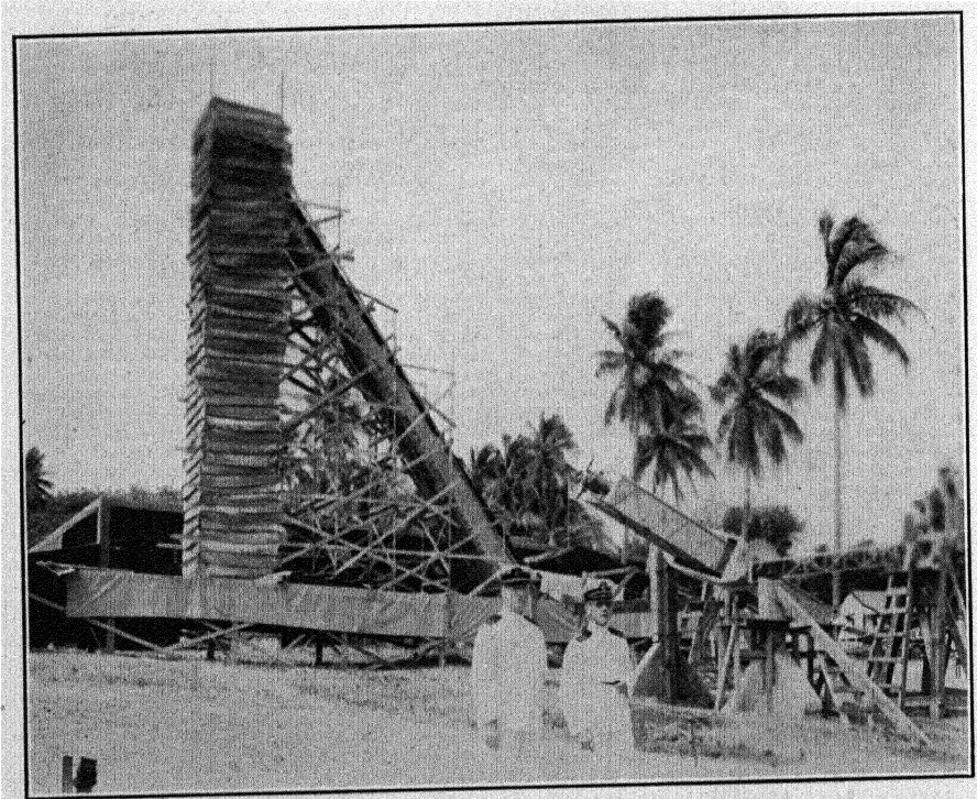
HUGE CAMERAS INSTALLED FOR THE 1930 ECLIPSE
