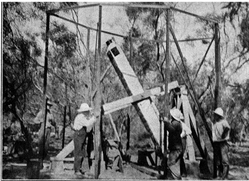
SAILORS OF THE AUSTRALIAN NAVY ASSISTING THEIR COUSINS FROM CANADA IN ERECTING THE EINSTEIN CAMERA
