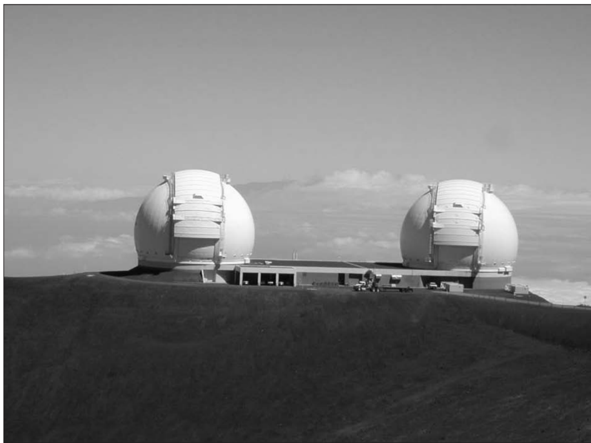
These two Keck telescopes at the top of Mauna Kea, Hawaii, can be linked together to form the Keck Interferometer, the world's most powerful ground-based optical telescope. (NASA/JPL)
