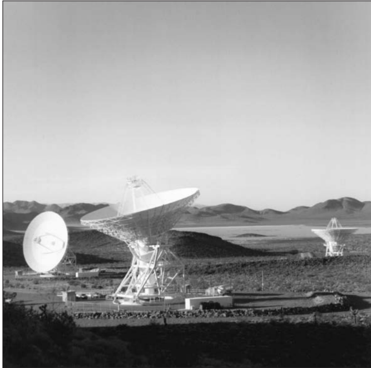
A long view of several of the radio dishes at the Goldstone complex, one of the three complexes that form the Deep Space Network (DSN). This system uses very long baseline interferometry to resolve radio signals received around the world. Radio telescopes kilometers apart can be linked together, forming the equivalent of a giant collector equal to that distance and hence providing higher resolution. The other complexes in the DSN are located near Madrid, Spain, and Canberra, Australia. (NASA)
