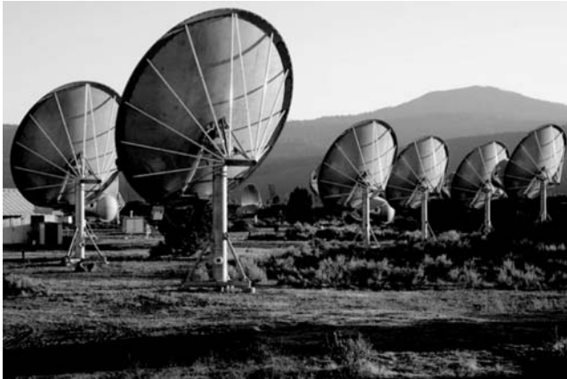
Figure 9.4 An artist's impression of the Allen Telescope Array. When it is completed, the telescope will consist of 350 dishes and will be the first telescope whose main purpose is to look for radio signals from extraterrestrial life (reproduced courtesy of SETI Institute).
