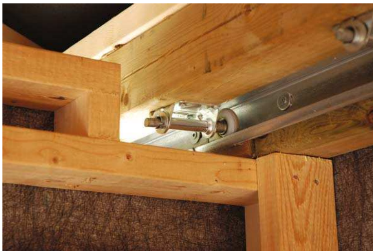
Figure 1.21. “The Ussher Observatory” – close-up of garage rollers and track. (Courtesy of Terry Ussher).
