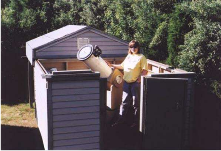
Figure 1.8. Gerald Dyck’s low observatory wall design with Dobsonian telescope inside. (Courtesy of Gerald Dyck) (See Color Plates).
