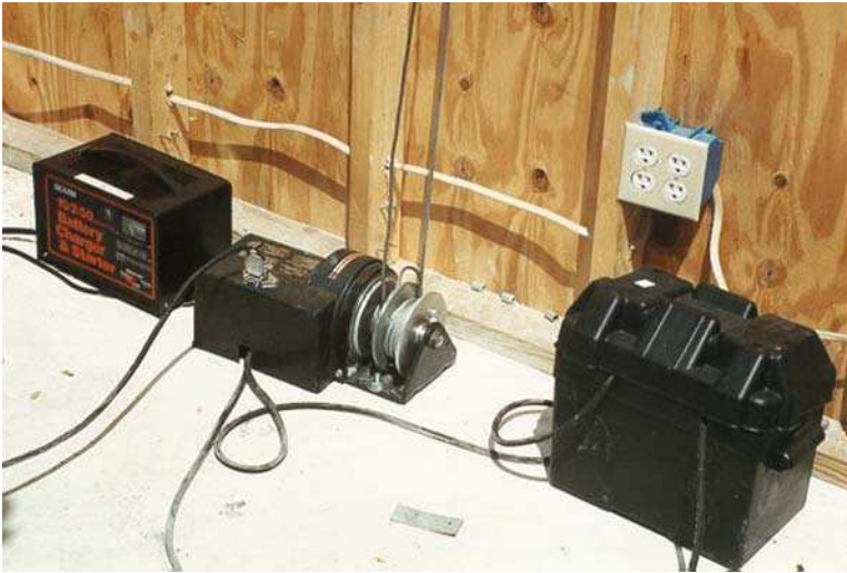
Figure 12.2. Motorized winch system operating on a 12 v battery. (Photo from the collection of John Hicks).
