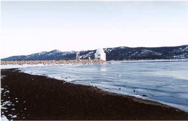
Figure 2.7. Big Bear Observatory on a man-made peninsula, Big Bear Lake, California, benefits from a laminar flow of air across a lake surface, high altitude, and a surrounding coniferous forest – all the necessary conditions to improve seeing. (Photo by John Hicks).
