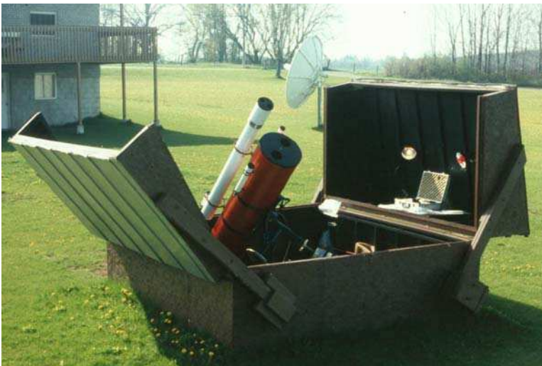
Figure 1.38. Paul Smith's (1995) Clam Shell Observatory open showing 10 in. reflector. Note that the north roof half swings only vertical affording an excellent shelf for equipment cases, lenses etc. (From the collection of John Hicks).
