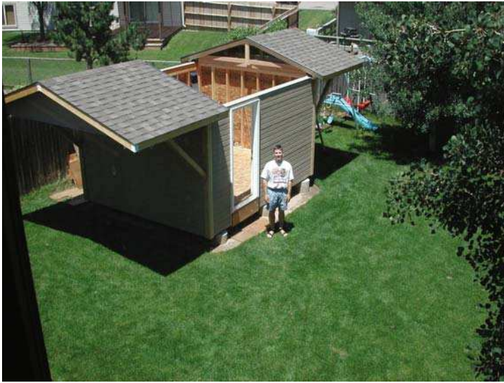
Figure 1.22. "Rocky Plains Observatory" – a twin roll-off roof observatory showing open roofs. (Courtesy of Bob Luffel) (See Color Plates ).
