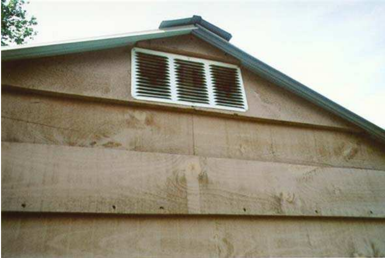
Figure 11.4. Photo of gable vent on Ussher Observatory. (Courtesy of Terry Ussher).
