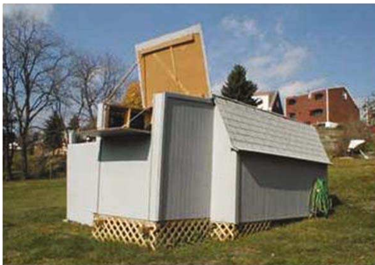
Figure 1.35. Barn-Shed style Observatory “Big Woodchuck Solar Observatory” showing the roof hatch open ready for observing. (Courtesy of Larry McHenry).
