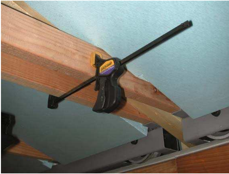
Figure 1.24. Roof Clamps hold the two halves together when the observatory is not in use. (Courtesy of Bob Luffel).
