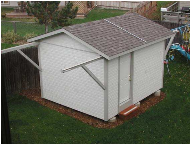
Figure 1.23. "Rocky Plains Observatory" – showing roofs closed and the gantry braces. (Courtesy of Bob Luffel) (See Color Plates ).
