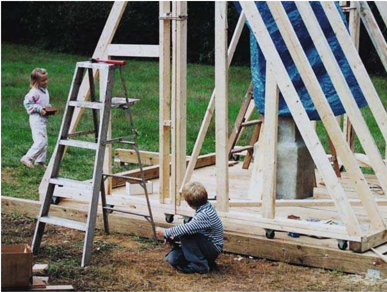
partially framed roll-apart observatory-showing casters
