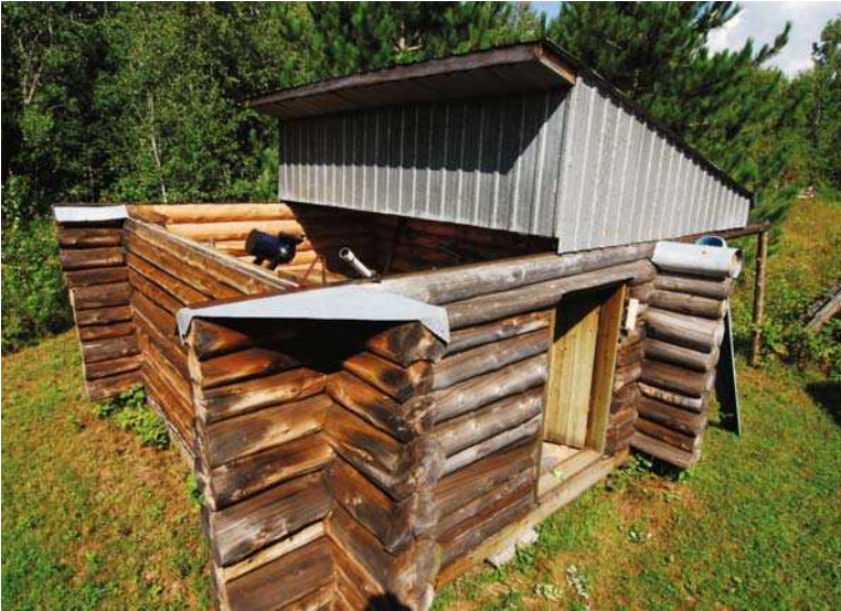
Figure 1.14. Log frame observatory with roof in open position. (Courtesy of Guy Boily) (See Color Plates).
