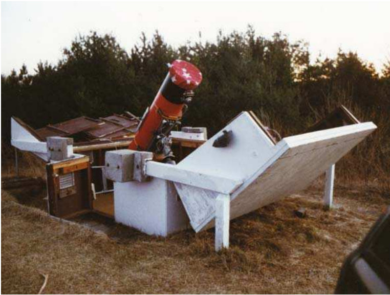
Figure 1.36. North York Astronomical Association Observatory at the “Bog” with roofs open showing the small entry door and excavated channel alongside wall for the swing of the counter – weights. (Courtesy of Danny Driscoll and NYAA).
