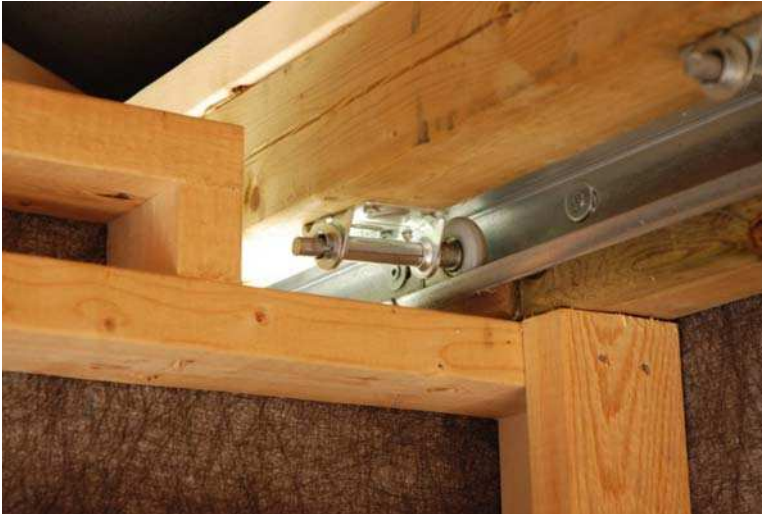
Figure 8.7. Photo – Terry Ussher’s “Sky Shed” Observatory showing garage door track and rollers on double plate under roof. (Courtesy of Terry Ussher).
