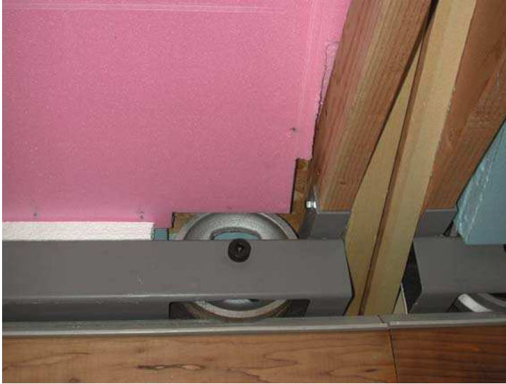
Figure 1.26. “Rocky Plains Observatory” inside track – illustrating how snugly the roof joists and thus the roof hugs the top of the observatory wall. (Courtesy of Bob Luffel).
