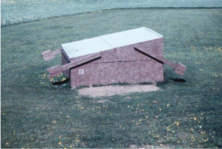
Figure 1.37. Paul Smith's Clam shell Observatory closed showing slope on split roofs. (From the collection of John Hicks).
