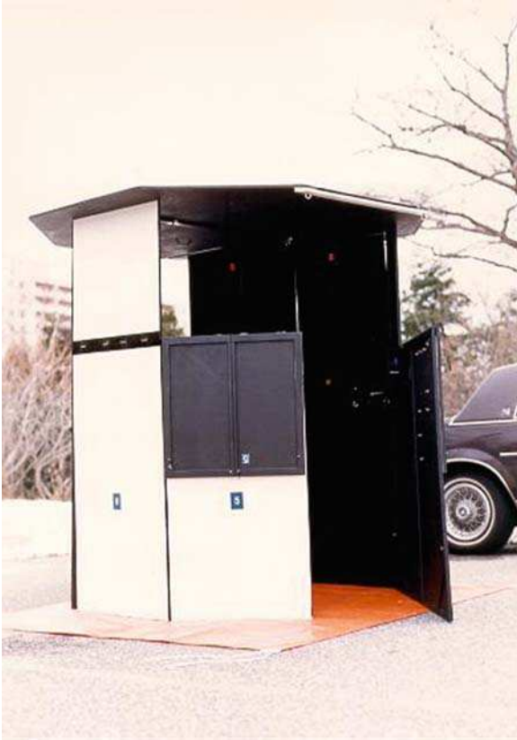
Figure 1.39. The first model of the "Clapp Trapp" showing the numbered wall panels, with some wall faces swung down, and the roof in place. The purpose of the wall panels which swung down was to observe objects nearer to the horizon. Not all wall sections had swinging panels in order to maintain stability. Too many panels swinging down would leave the roof unsupported. (Courtesy of Doug Clapp).
