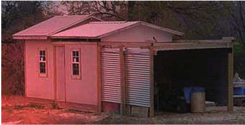
Figure 1.29. “Ballauer Observatory” – illustrating higher warm room section, lower roll-off roof, and attached open storage area. (Courtesy of Jay Ballauer).
