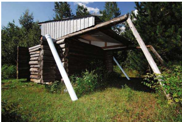
Figure 1.17. Log frame observatory gantry. (Courtesy of Guy Boily).
