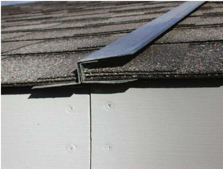
Figure 1.28. Z-flashing on closed roofs – “Rocky Plains Observatory.” (Courtesy of Bob Luffel) ( See Color Plates ).
