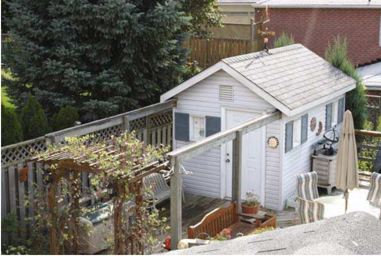
Figure 1.10. Petherick Roll-Off Observatory showing gantry transformed into trellis. (Courtesy of Dave Petherick) (See Color Plates ).
