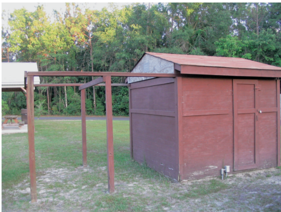
Plate 15. A typical roll-off roof backyard observatory.
