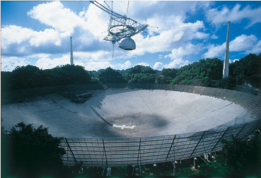
a Arecibo has the world's largest single-dish radio antenna, shown here, with a diameter of 305 meters (1000 feet).
