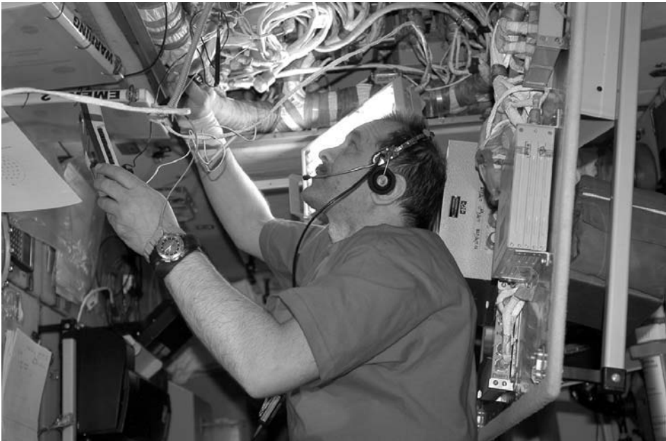
Figure 67. Expedition-13: Pavel Vinogradov works on the lighting inside the Pirs airlock.
