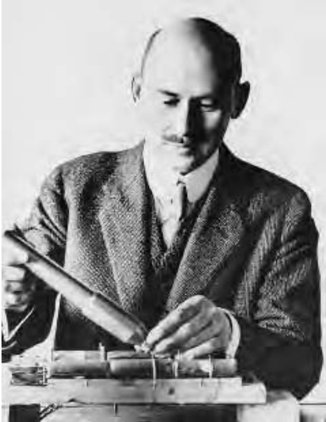
Dr. Robert H. Goddard, the reclusive genius who is widely acknowledged as the “father of American rocketry,” is shown with a steel combustion chamber and rocket nozzle in this 1915 photograph. (Courtesy of NASA)
