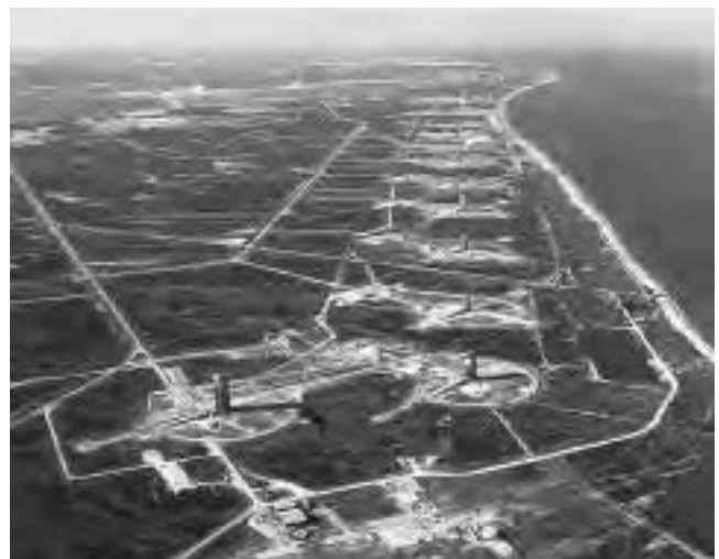
Looking north at the rocket launch complexes of Cape Canaveral Air Force Station in the early 1970s. During the ballistic missile race of the cold war, this unique collection of launch facilities, situated along the shore of the Atlantic Ocean in central Florida, became known as “missile row.” The Titan rocket launch complex (called Complex 40) appears in the distance. (Courtesy of NASA and the U.S. Air Force)
