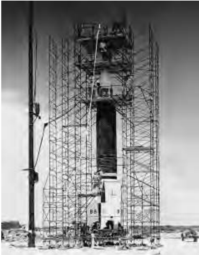
This historic photograph shows the construction scaffolding used to create a contemporary gantry at Cape Canaveral Air Force Station in July 1950 to help workers prepare the Bumper 8 rocket for launch. (Bumper 8, the first rocket shot from Cape Canaveral, was a captured German V-2 rocket modified by American rocket engineers.) (Courtesy of the U.S. Air Force)
