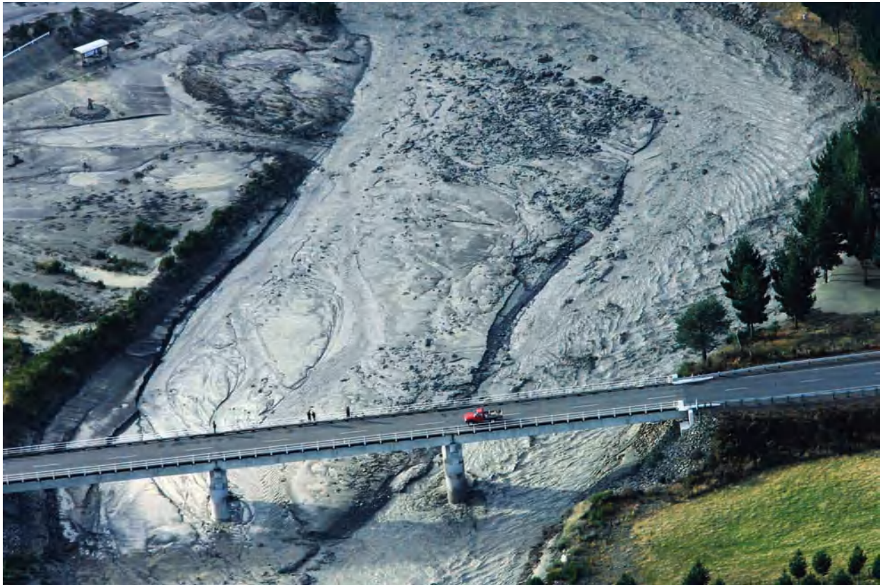
Mudflow on Whangaehu River after lahar from crater lake of Mount Ruapehu in the central North Island of New Zealand, March 18, 2007: The bridge over river is Tangiwai road bridge. (Anthony Phelps/Reuters/Landov)
