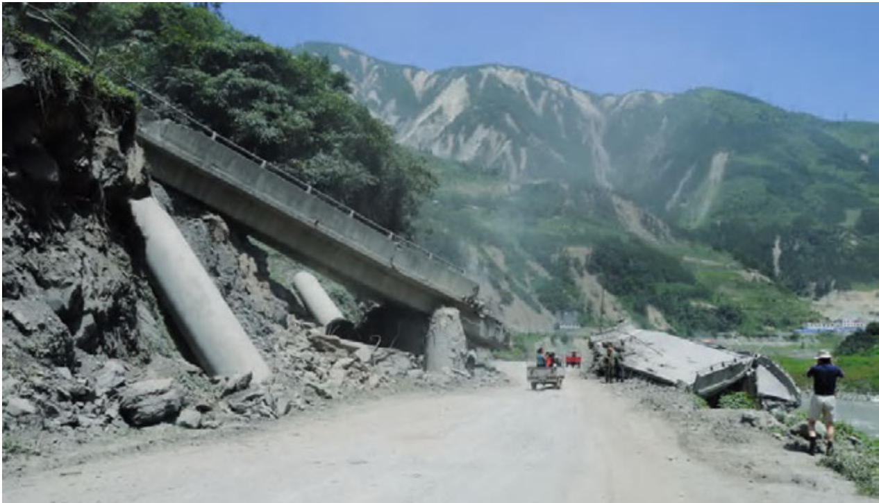
Damage from ground shaking and landslides in Yingxiu, Sichuan Province, China, from May 12, 2008, magnitude 7.9 earthquake (T. Kusky)
