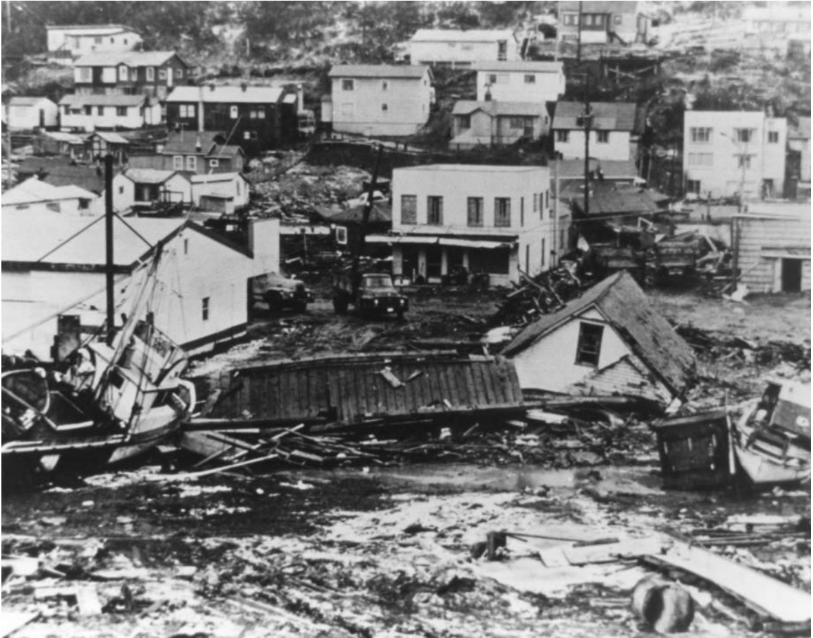
Figure 129 Tsunami damage at Kodiak from the 1964 Alaskan earthquake.
