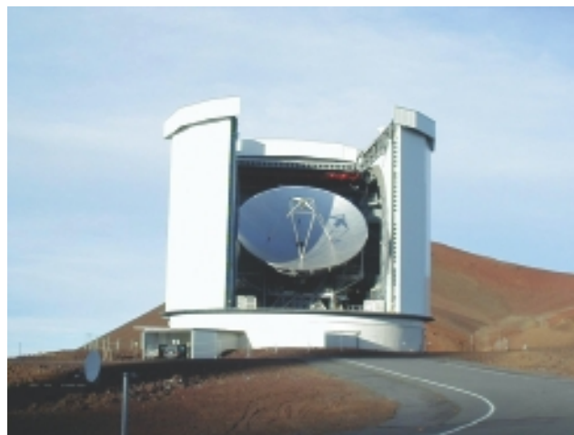
Figure A.4 A rare view of the James Clerk Maxwell Telescope after the telescope membrane had been removed in preparation for removing the secondary mirror unit. Credit: James Clerk Maxwell Telescope, Mauna Kea Observatory, Hawaii.
