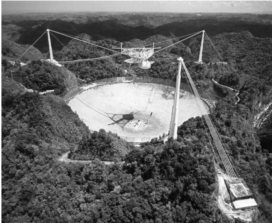
Figure 21.19. The 1000 ft radar-radio telescope (Cornell University) at Arecibo, Puerto Rico. (By courtesy of the NAIC-Arecibo Observatory, a facility of the NSF.)
