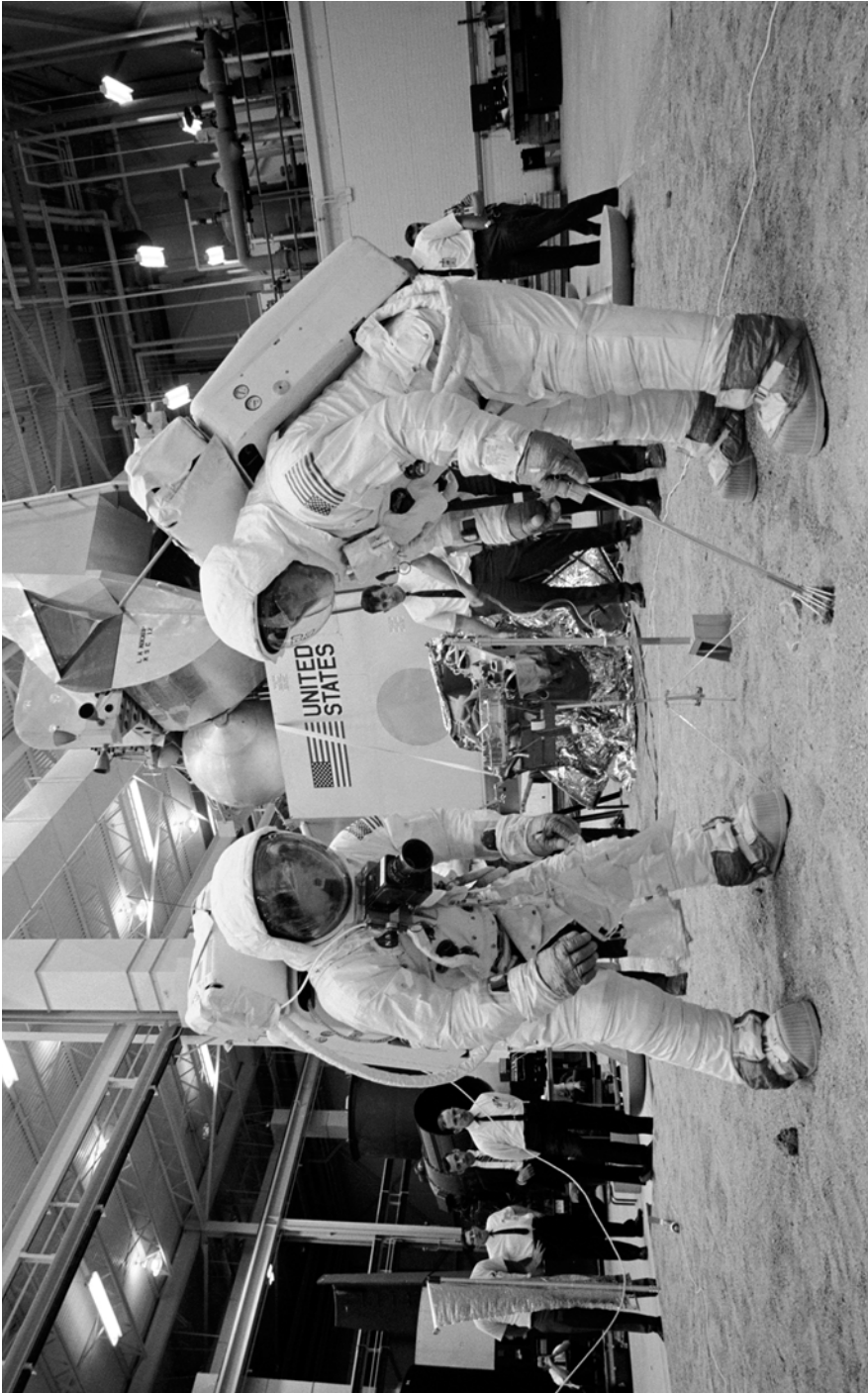
Neil Armstrong and Buzz Aldrin rehearse 'documented' (photographed) sampling using tongs, a gnomon and individual sample bags.
