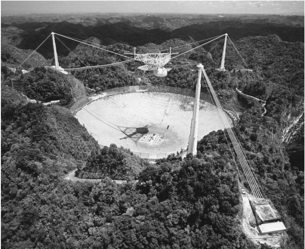
The Arecibo Observatory is the world's largest radio/radar telescope. The facility, located in a large, bowl-shaped natural depression in the tropical jungle of Puerto Rico, has a diameter of 1,000 feet (305 m). (NASA)
