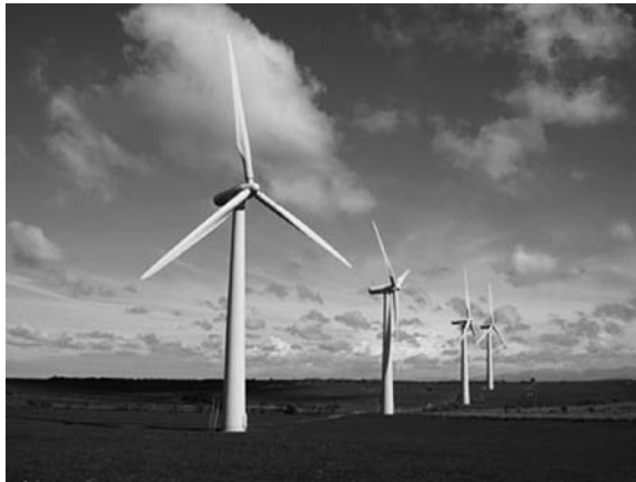
Figure 1.1 Modern utility-scale wind turbine. Reproduced by permission of General Electric
