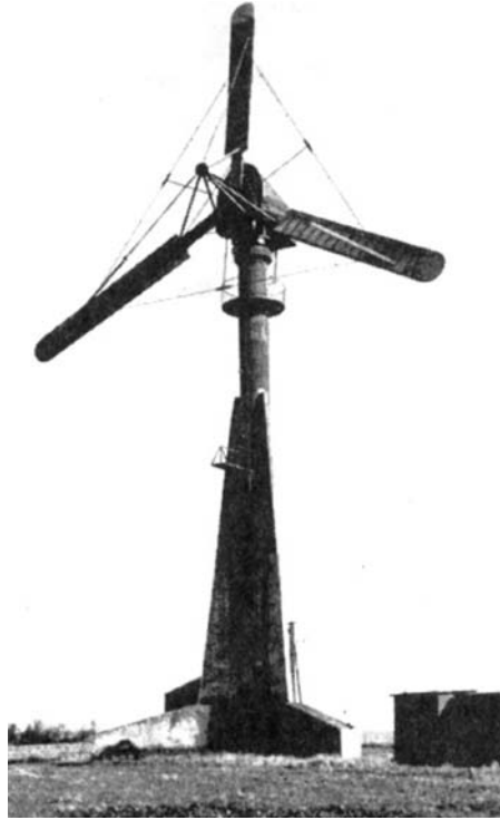
Figure 1.15 Danish Gedser wind turbine. Reproduced by permission of Danish Wind Turbine Manufacturers
