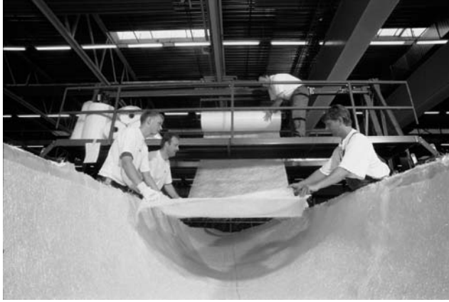
Figure 6.20 Laying fiberglass cloth into blade molds. Reproduced by permission of LM Glasfibre
