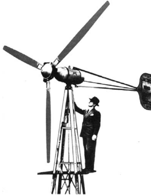
Figure 1.14 Jacobs turbine (Jacobs, 1961)
