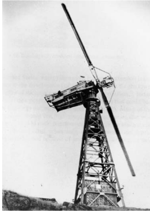
Figure 1.16 Smith–Putnam wind turbine (Eldridge, 1980)
