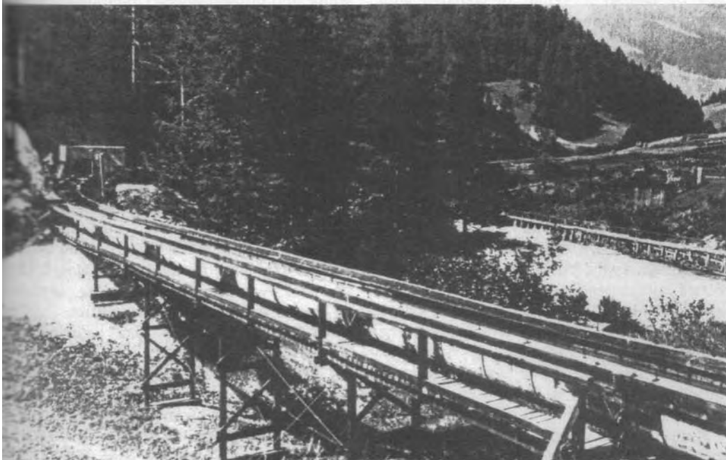
Fig. 12.4 Schauberger's log flume followed the contours of the valley
