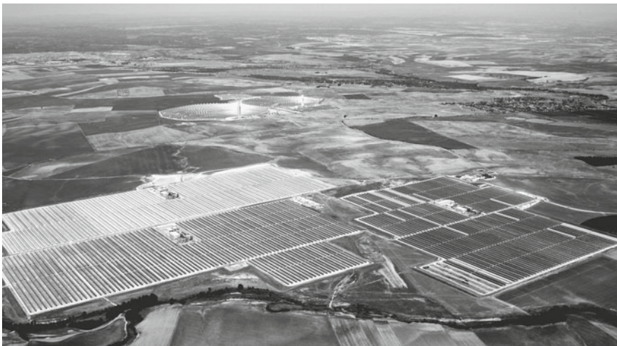
The Solnova Solar Power Station near Seville, Spain. (Credit: Abengoa Solar, via Wikimedia Commons.)
