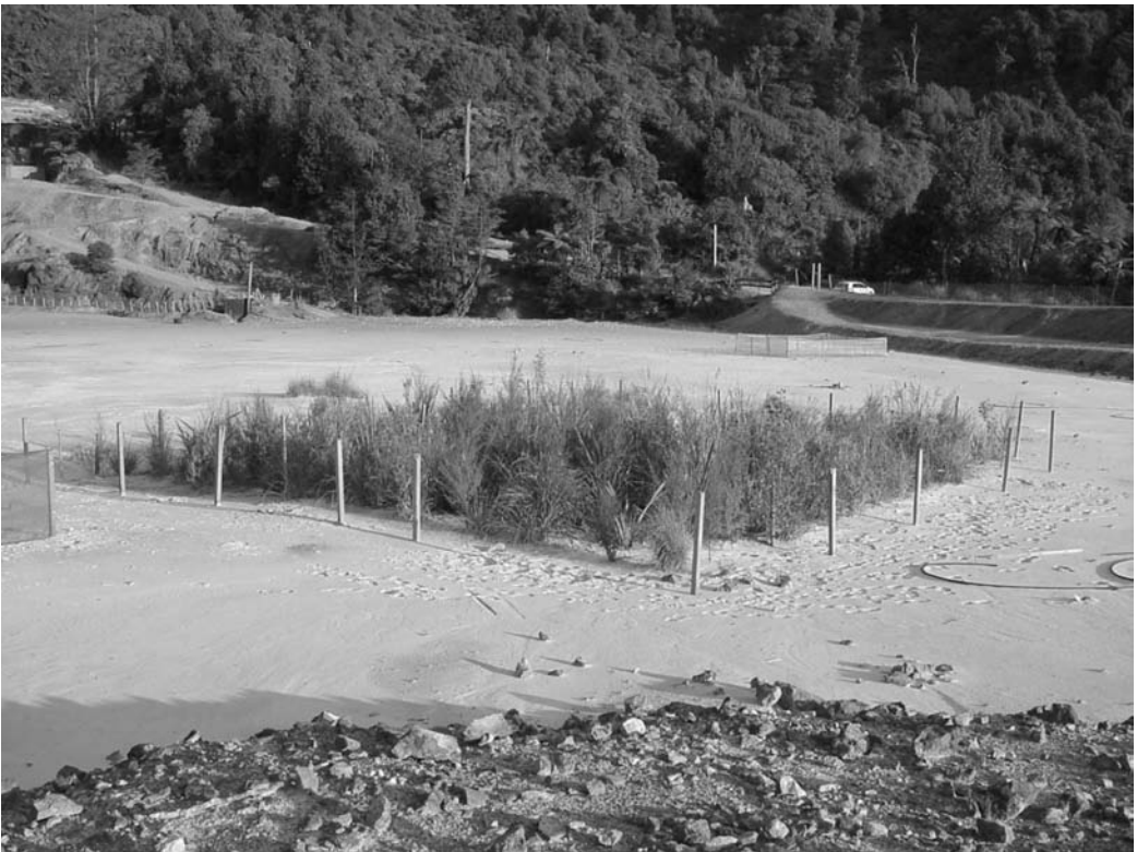
FIGURE 6.4 Vegetation established on the Tui mine tailings, Te Aroha, New Zealand. The vegetation has reduced metal mobility by adding organic matter to the substrate and returning some rainfall to the atmosphere via evapotranspiration.
