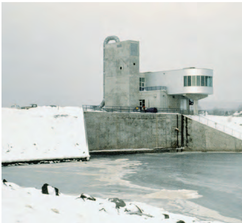
Annapolis Royal Tidal Generator, a hydroelectric power station in Nova Scotia, is located in Annapolis Royal by the Bay of Fundy, home of the world's highest tides. Twice a day, the tide comes in and out. Twice a day the turbine turns. Twice a day electricity is generated and supplied to the provincial electric grid. Stephen J. Krasemann/Photo Researchers, Inc.
