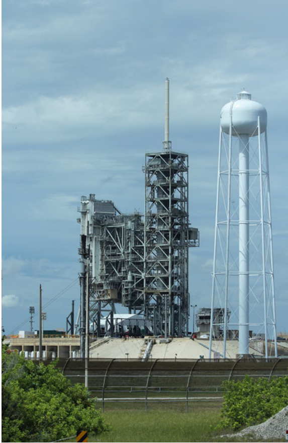
Fig. 2.32 Launch Pad 39A at the Kennedy Space Center. A total of 12 Saturn V and 81 Space Shuttle flights launched from here. It is currently used by the Falcon 9 and Falcon heavy rockets. The concrete ramp leading up to the launch platform, with its 250 m length and a slope of 5% allows rockets to be delivered upright on a crawler. The flame trench under the platform (not visible in this photo) is 13 m deep, 18 m wide and 137 m long. The water tower for the cooling system is 88 m high. The pad has undergone modifications to accommodate vehicles by SpaceX (Image: B. Ganse)
